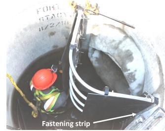
14) Attach both side sheets at wall using (2) fastening strips and provided screws. Use hand clamps for assistance. Apply pressure and adjust your drill's torque setting to prevent stripping.
