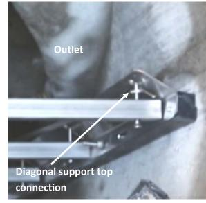
12) Remove nut from lower arch adjusting bolts (each side). Attach bottom of diagonal support at this location, on each side.
