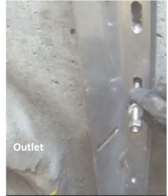
10) Working from the bottom up and leaving nuts and bolts loose, attach arches to wall brackets. Go to next step prior to attaching top arch.
