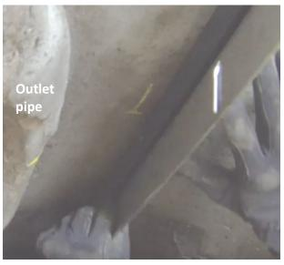
8) Align wall bracket with marks made in Steps 5, 6 and 7. Use level to ensure bracket is vertical prior to next step.
