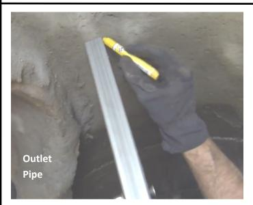
5) Mark wall at outside edges of arch assembly. Remove arch assembly and adjust all remaining arch assemblies to match.
