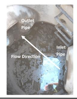
4) Hold arch assembly horizontally at center of outlet, applying inward pressure toward the pipe. Adjust arch assembly to avoid obstructions and allow room for installation.
