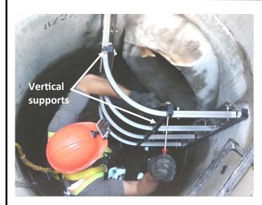
13) Attach vertical supports. Tighten all nuts and bolts on skimmer structure, working from center of skimmer towards the walls.
