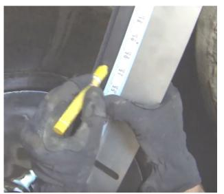
7) Measure and mark the center of the wall bracket on the back (pipe side) edge.
