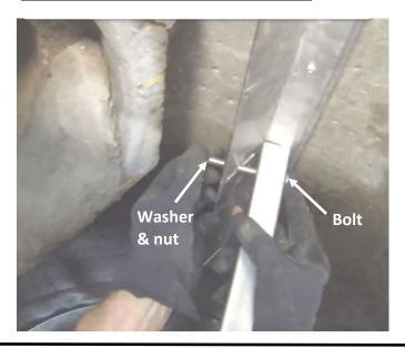
11) While installing top arch, attach diagonal supports between arch and wall brackets.
