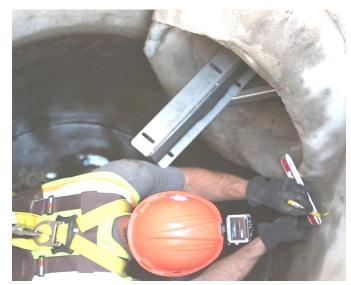
6) Make horizontal marks at center of outlet pipe, crossing bracket marks from previous step.
