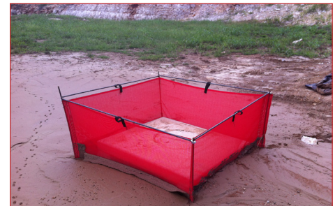
"Big Red AI Protector with 4" sediment load after initial Rain Event.
