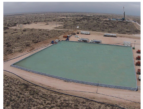
Primary & Secondary Containment
