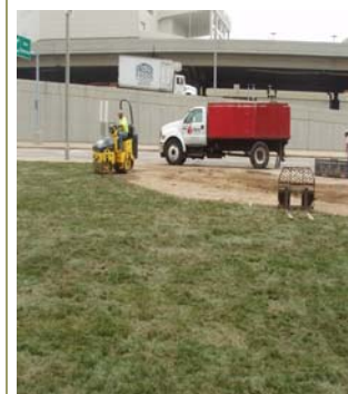
A final look at the finished product
