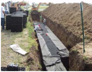
Raintanks being installed in excavation site
