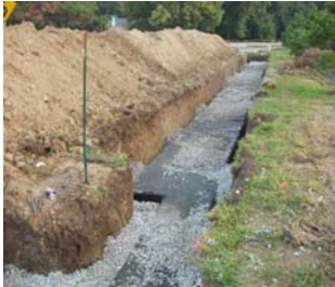
Raintanks are installed with the beginning of the cover up
